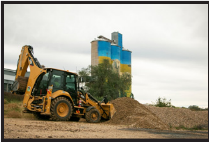
Works at Hacketts Ln (near the Merriwa Silos).
